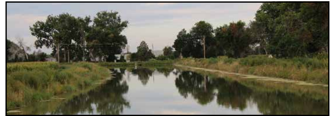
This is a recharge pond project of the North Platte NRD. It gets filled with surface water from the Enterprise Irrigation District, with temporarily leased water rights.
